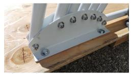
Secure frame to plywood using 1.5" bolts, washers and nuts
