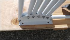
Add a Speedway Shelters Diamond Locate 2 each anchor holes on both sides of frame assembly. Mark and drill holes
